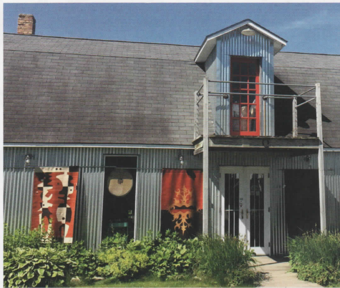
The Martínezes turned a two-story garage into their studio gallery. Many of the area's craft venues are housed in refurbished buildings.
